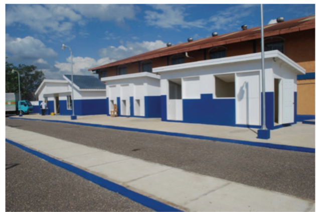
The Linstead Transportation Centre, after the construction works.
